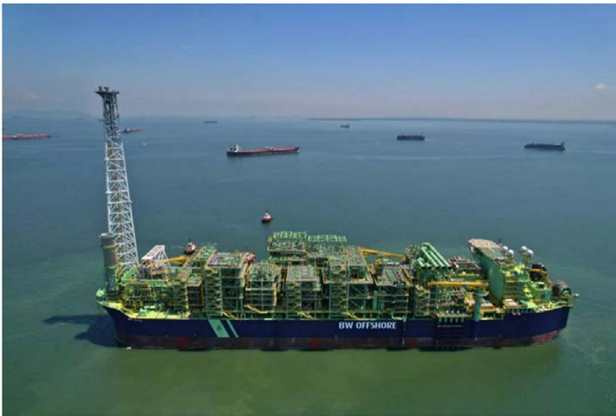
Successful delivery of FPSO BW Opal to BW Offshore
